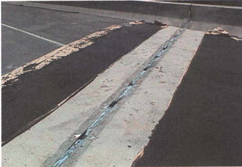
RAISING JOINT FOR NEW A.C. OVERLAY WITH SEAL
