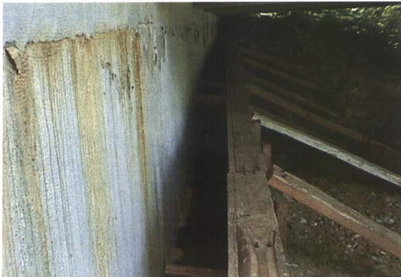
UNFINISHED WORK @ ABUT-2 FORMS IN PLACE
