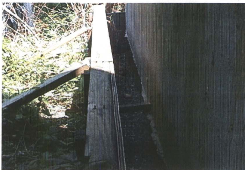
UNFINISHED WORK @ ABUT-2 FORMS IN PLACE
