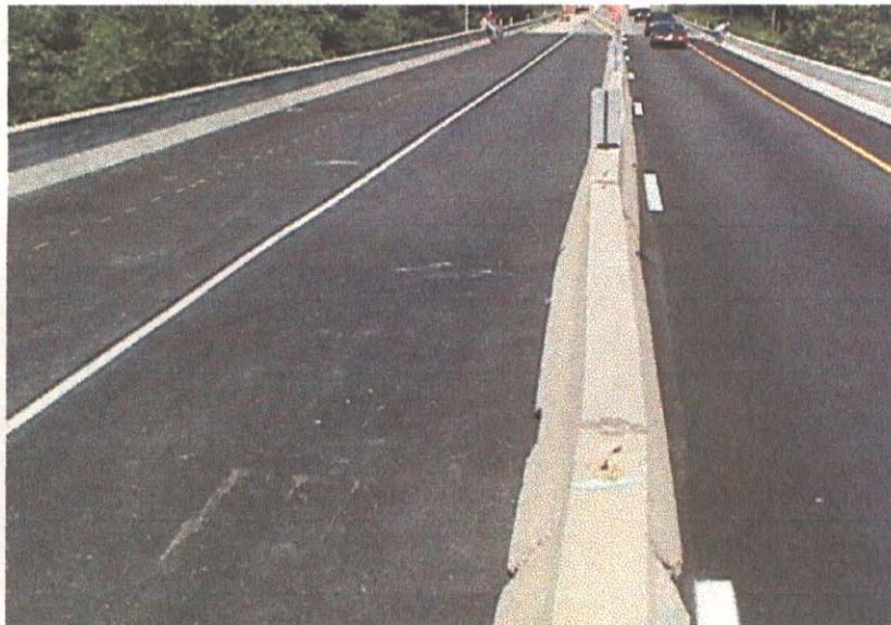
ACROSS TOP OF DECK
