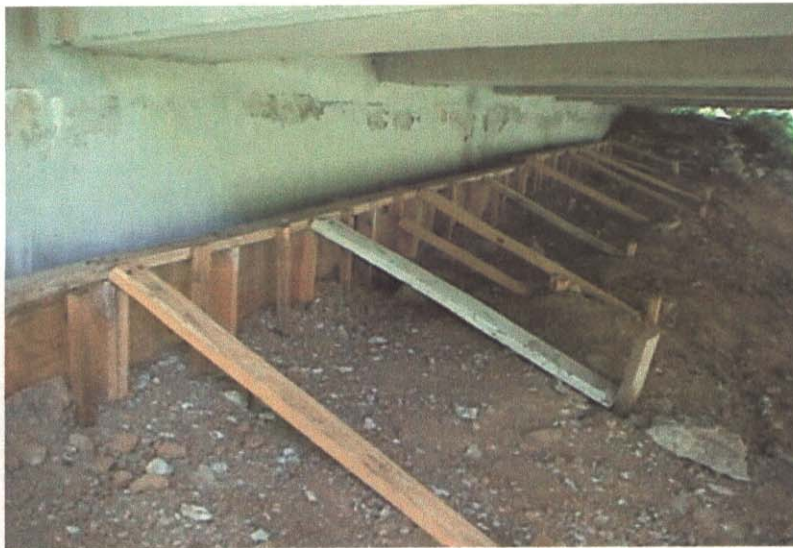
CURTAIN WALL SETTLEMENT REPAIR AT ABUTMENT #2
